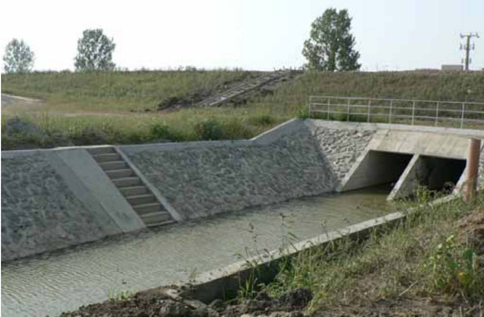
Figure 5.3: Construction of the outlet of the first retention reservoir
